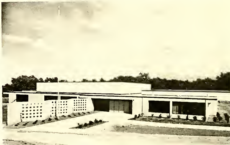
R. Brown McAllister Elementary School, completed in 1958, one of the outstanding school plants in the State
